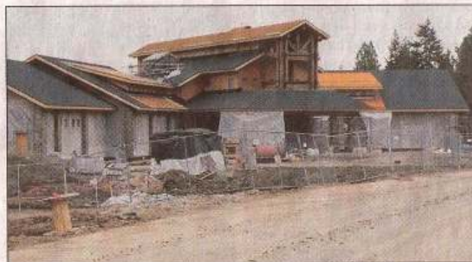
SWIFTWATER CELLARS WINERY on Roper Rider Golf Course, Suncadia, is nearly closed in. The $10M project required 3,400 cubic feet of concrete, much of which will be grained and stained to look like wood.
