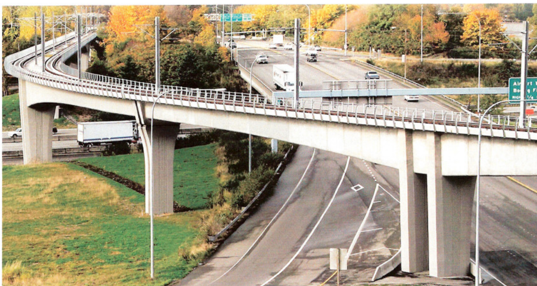
Photo courtesy of International Bridge Technologies Inc.
